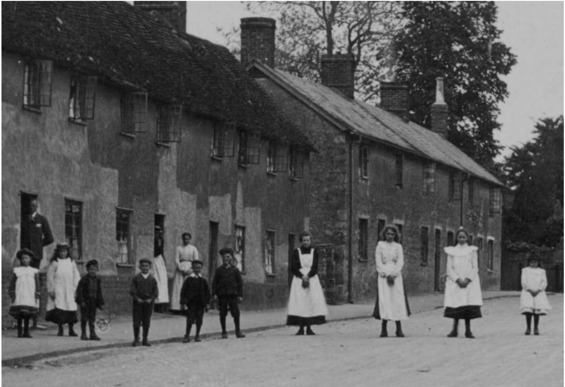
High Street facing north: 39-44 Bletsoe (now demolished) at right / rear, 33-35 Bletsoe at left. Single view at top is CRO 6498 c1900 by Sweetland. Other two are details.
