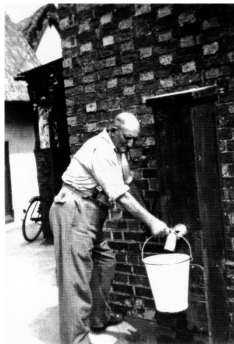
Pump at 29 Bletsoe c1960
