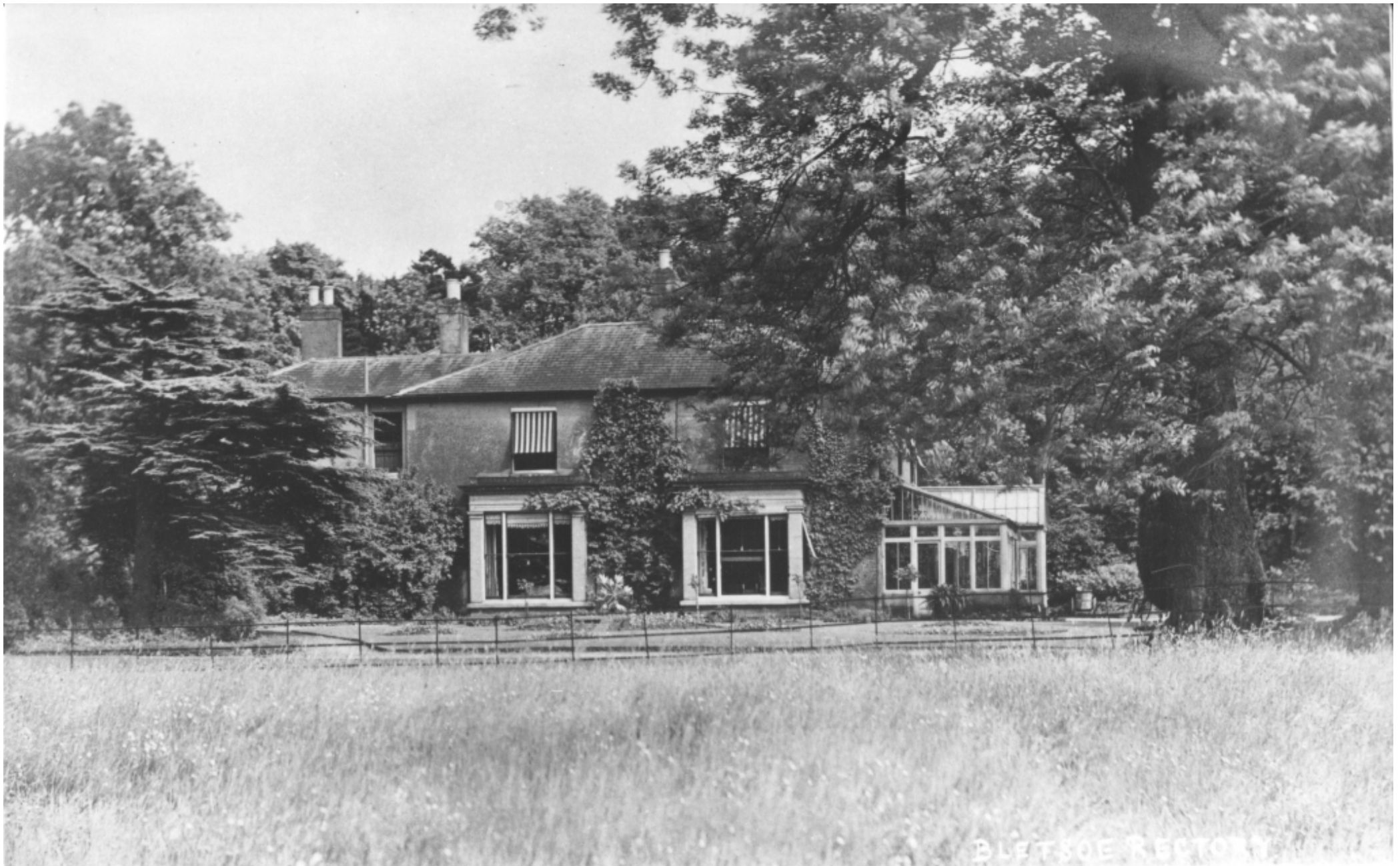
Bletsoe Rectory from the west, c1906
