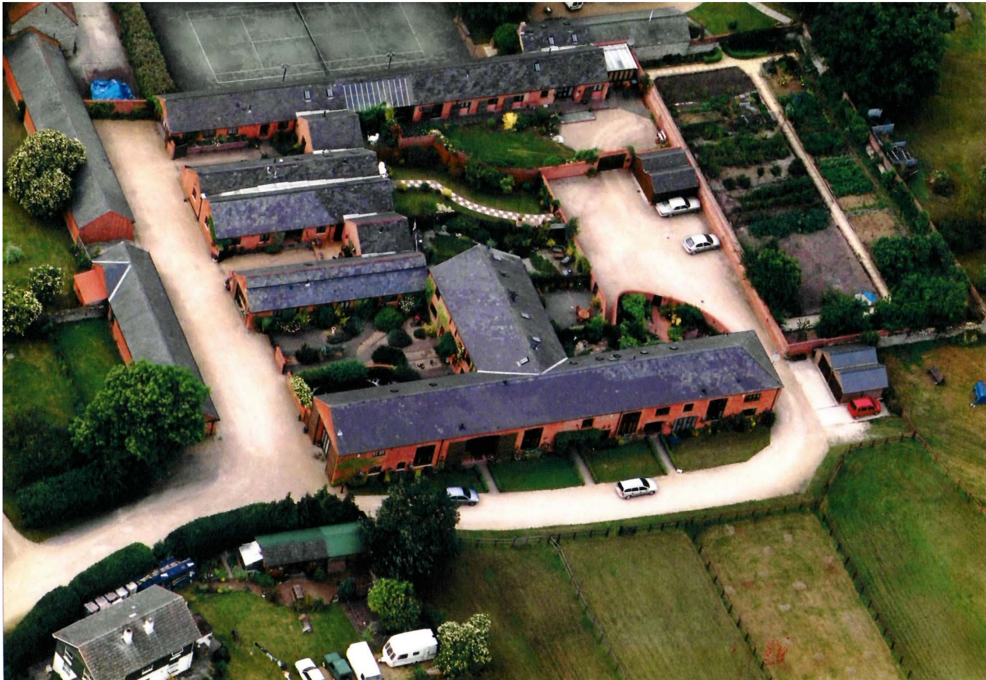
Castle Farm barns after 1990s residential conversion
