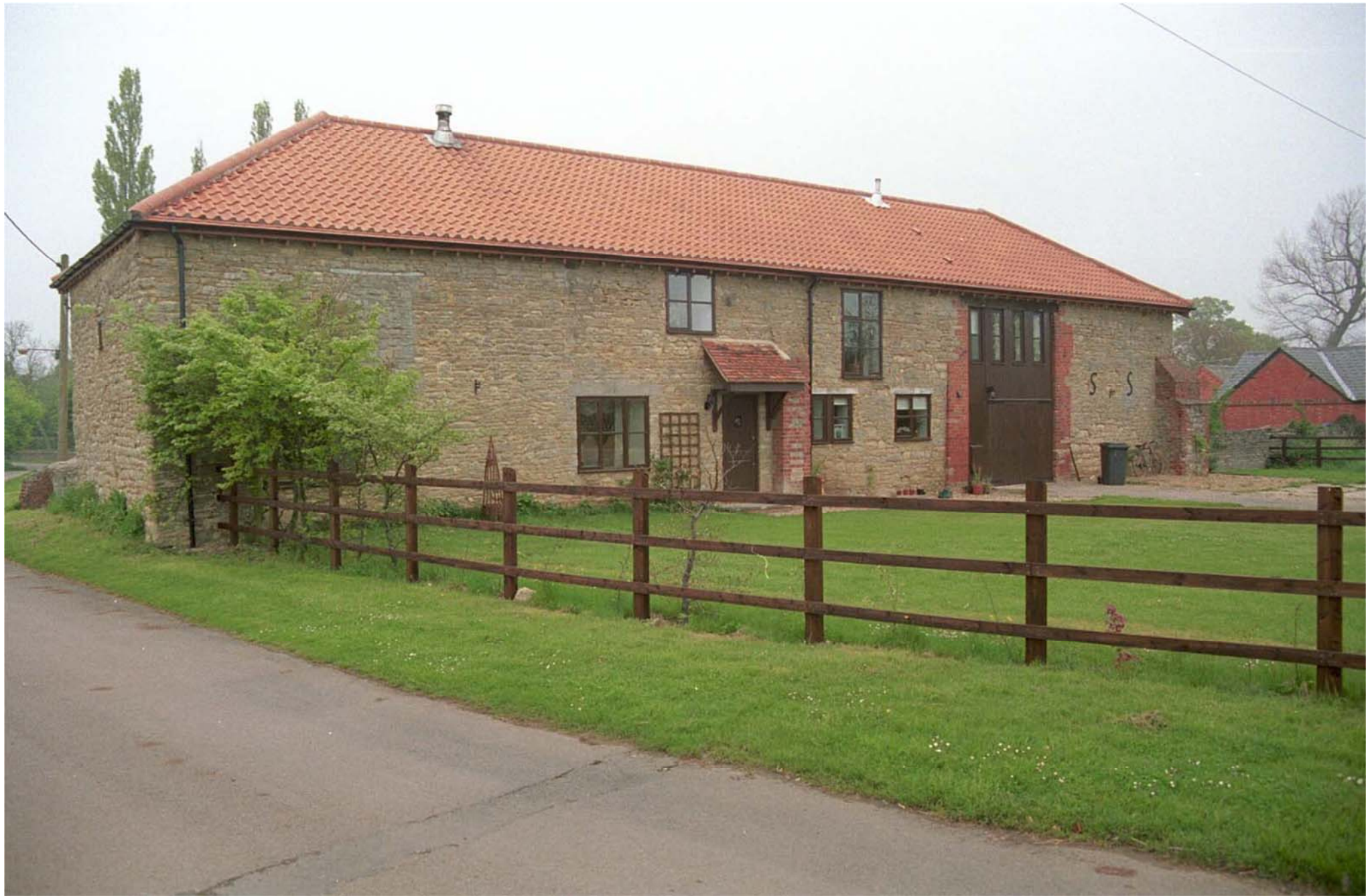
Barn at Castle Farm, Coplowe Lane
