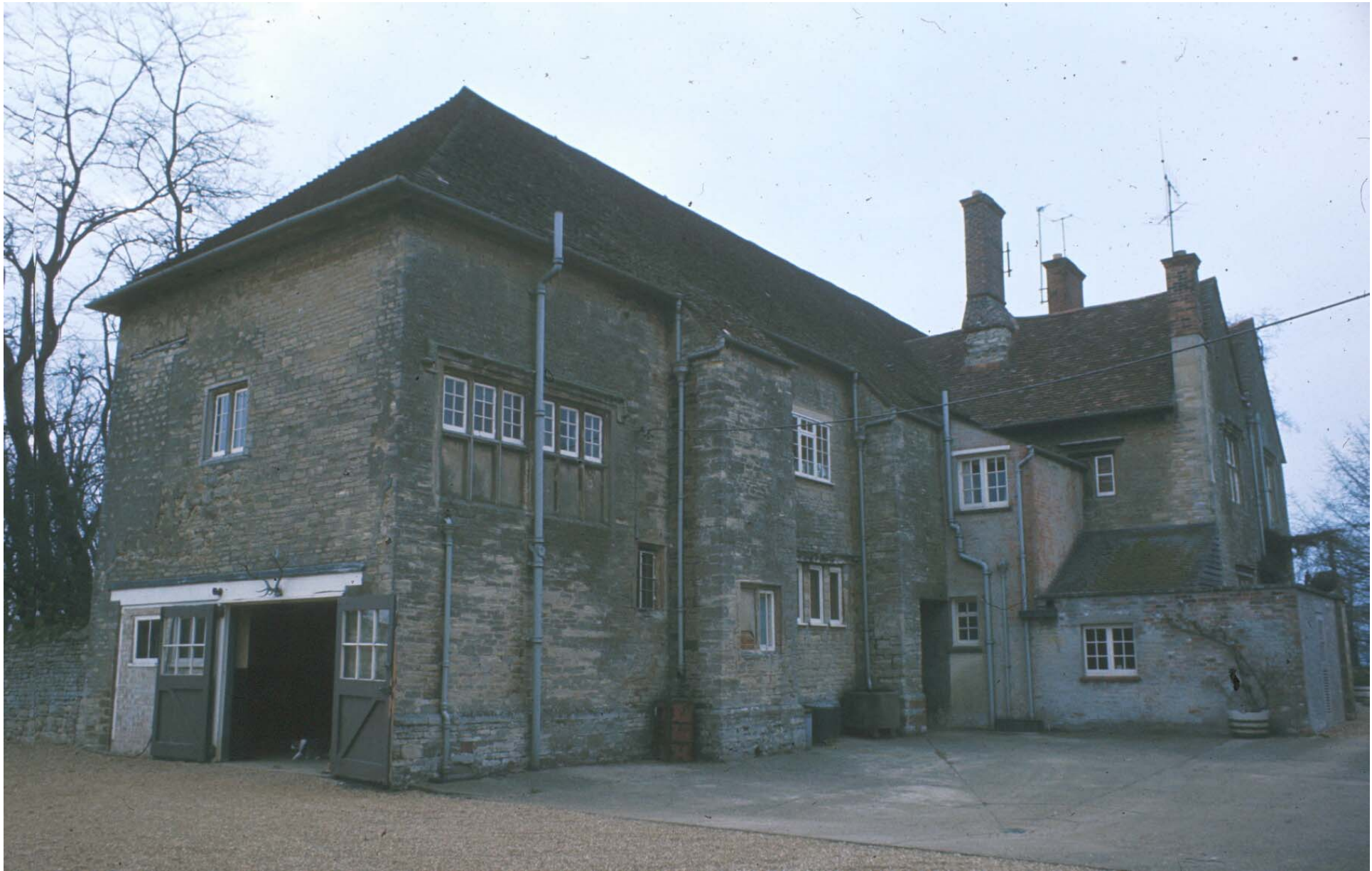
Rear and east side elevations 1980s
