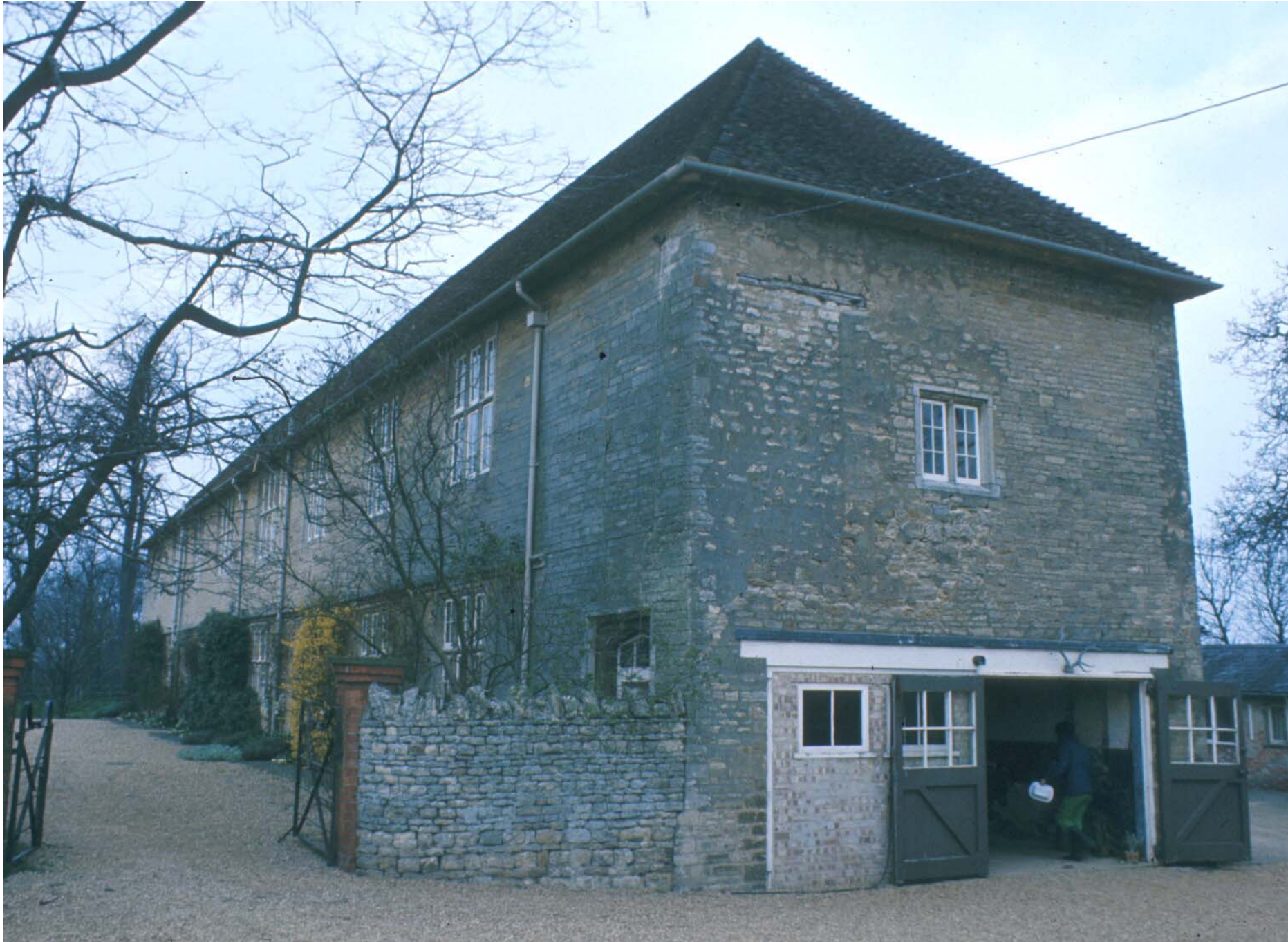
Front and east side elevations showing evidence for alterations c 1800 at time of reduction from three to two storeys, 1980s
