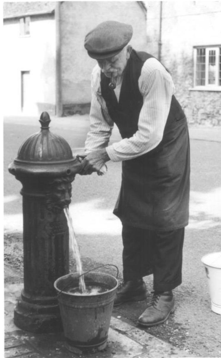
William Curtis drawing water c1955. Pictured at the standpipe outside St Mary's church and opposite his cottage at 44 Bletsoe. The majority of the cottages did not have piped water or any main sewerage until the 1960s. EB186 ( Mrs Daphne Waugh )
