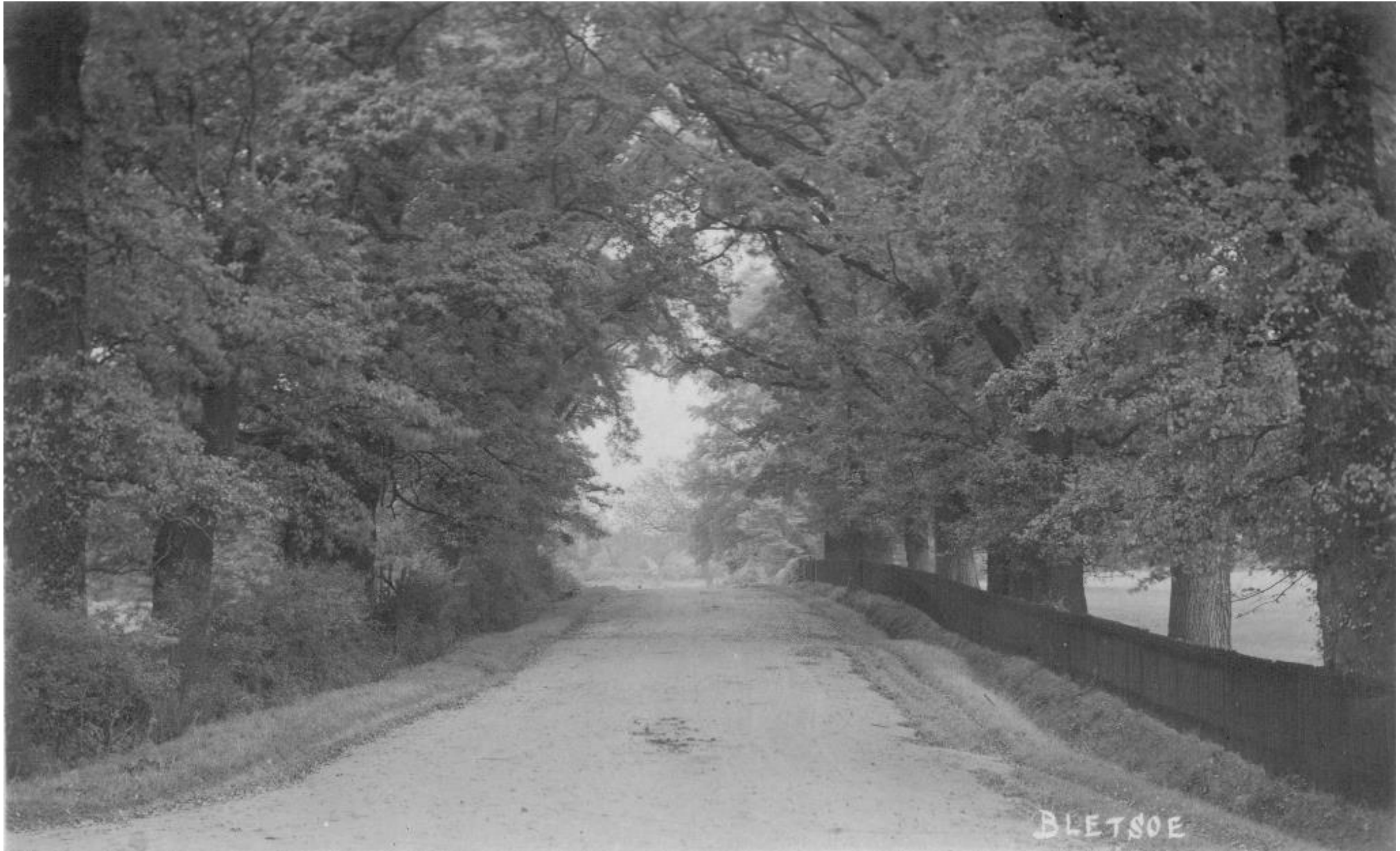
Bletsoe entrance looking in: c1905
