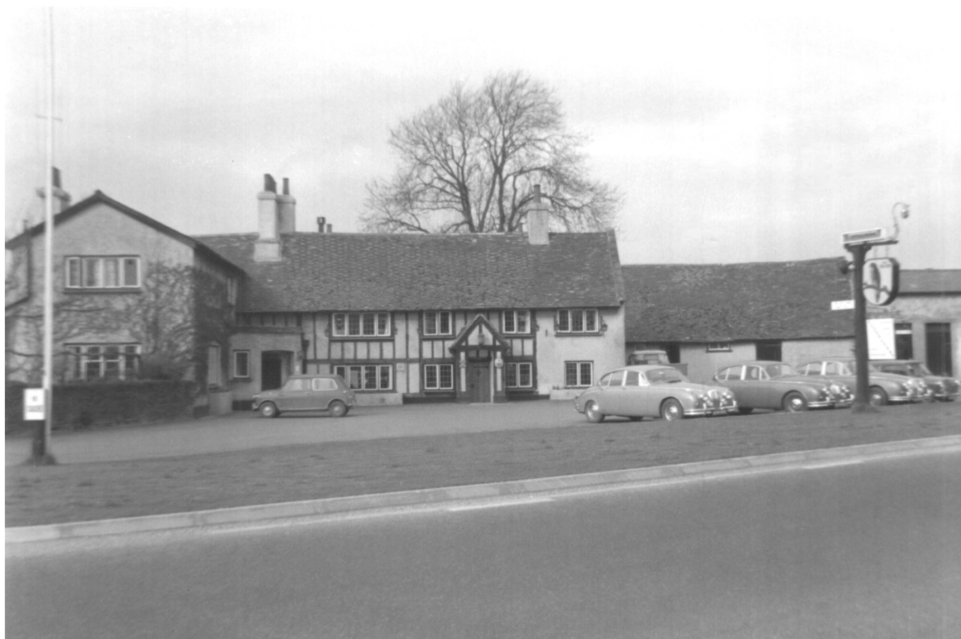
The Falcon Inn from the A6: above 1940s, below 1965
