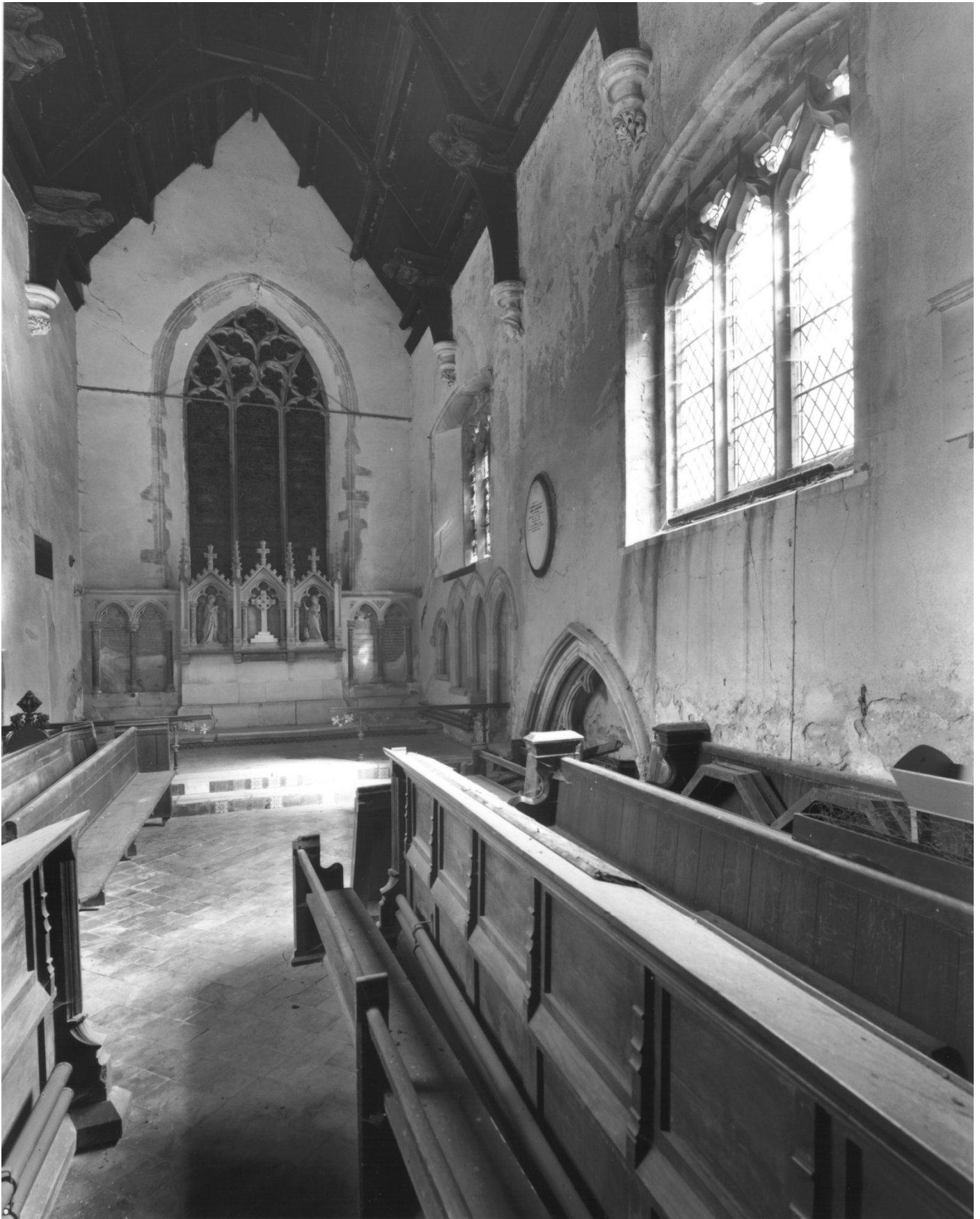
Chancel interior facing east, showing later removed choir pews 1975 when redundancy was a possibility (Beds CC Photographic Unit; Bedfordshire Archives Z50-18-6)
