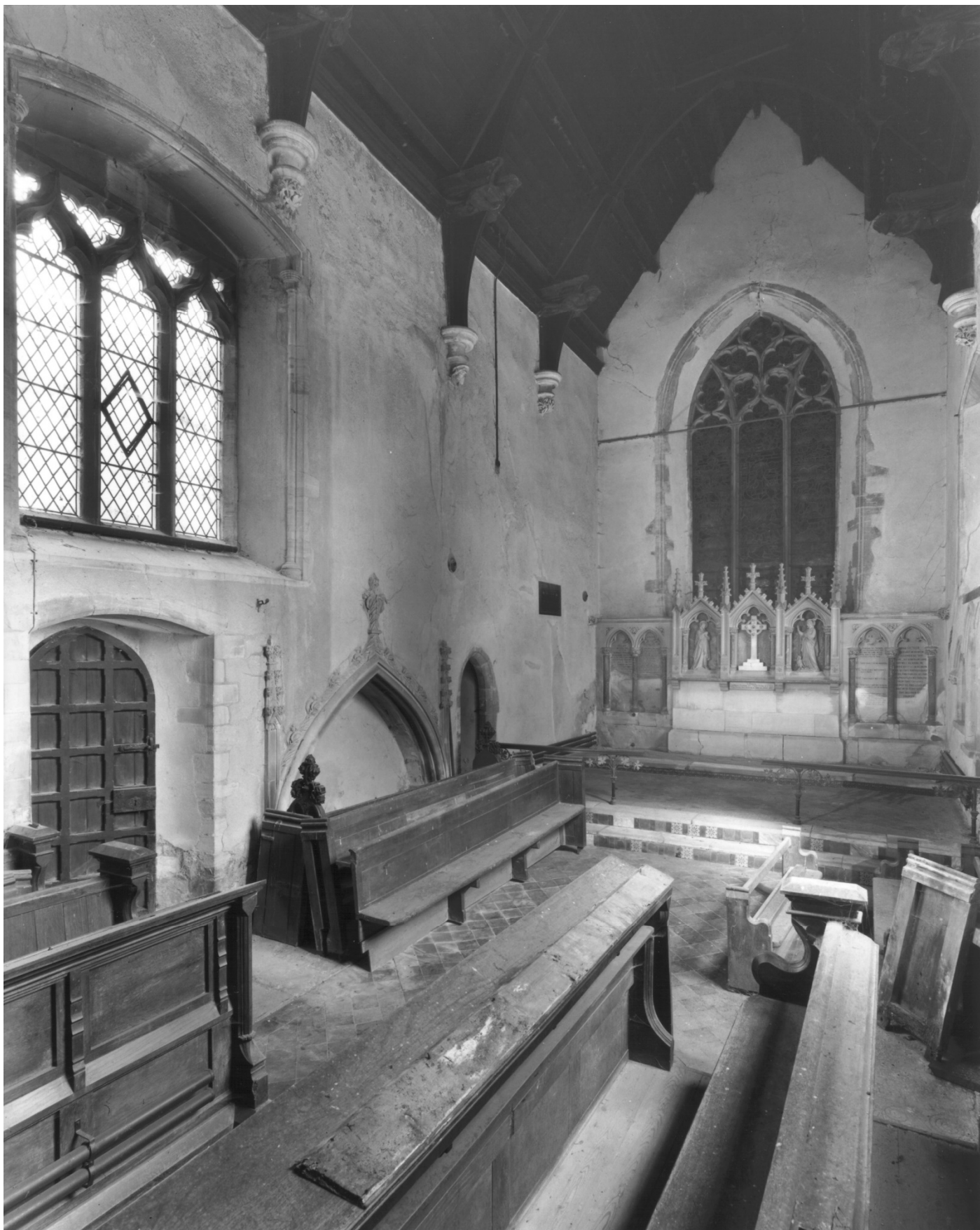
Chancel interior facing north-east, showing later removed choir pews 1975. when redundancy was a possibility
