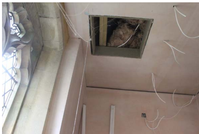
J Lined-out interior of old vestry > DDA compliant WC
