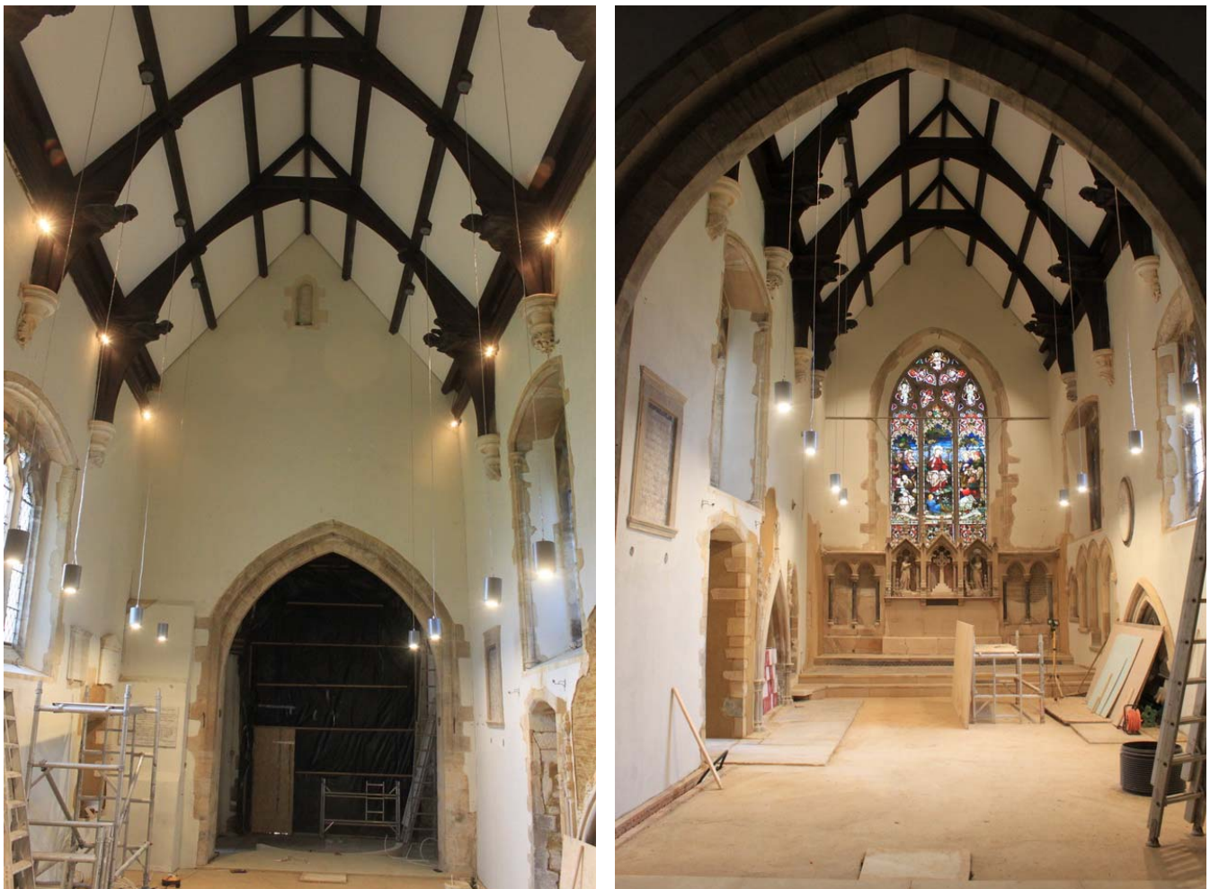
A B Chancel facing west ( left ) and east ( right ): scaffolding removed; lights in place
