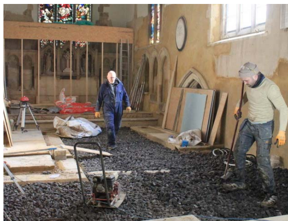
D Chancel facing east: make-up for limecrete floor finish
