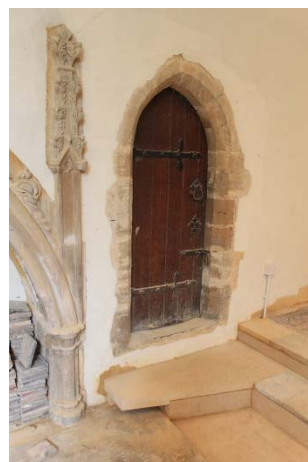
K Door to WC from chancel
