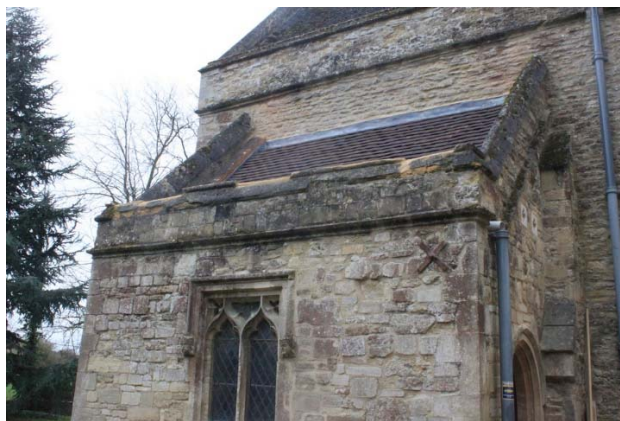
I Re-roofed vestry with mortar repairs to parapet
