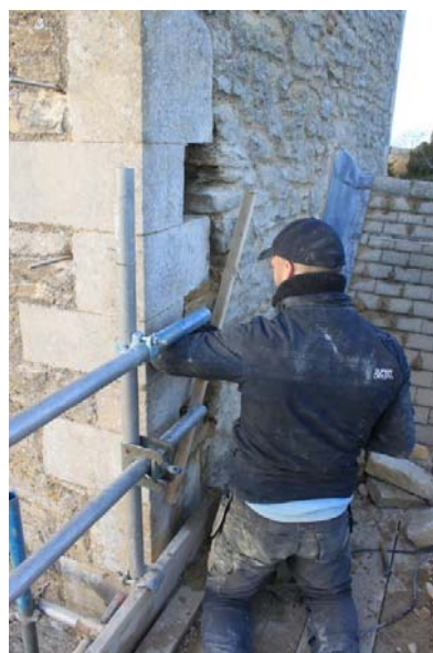
High-level external repairs: G left at junction of 1860s turret and chancel; H centre fixing across the crack between the (later) tower quoins with pins at left hand side; J right replacing poor quality stonework on the site of the crack
