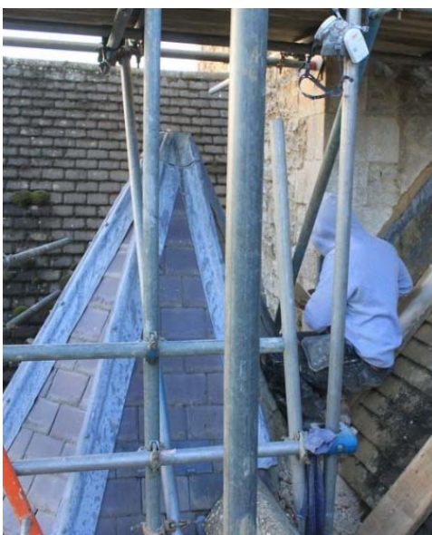
High-level external repairs: G left at junction of 1860s turret and chancel; H centre fixing across the crack between the (later) tower quoins with pins at left hand side; J right replacing poor quality stonework on the site of the crack
