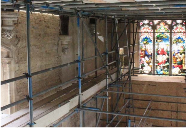
C D High-level wall plaster renewal. Left showing defective area stripped at left; right wet replacement lime plaster
