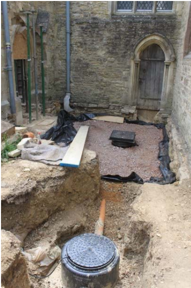
K Pumped drainage from north side of chancel L The other end - 'invisible' sewer connection in Coplowe Lane
