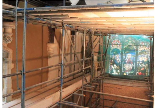
C D High-level wall plaster renewal. Left showing defective area stripped at left; right wet replacement lime plaster
