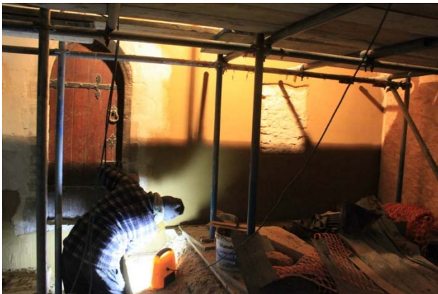
Re-plastering: E left north wall showing blocked ambry at right centre; F right south wall sedilia with top coat within niche seats arches, piscina at left; at extreme right base-coat plasterwork scratched with key for application of top coat
