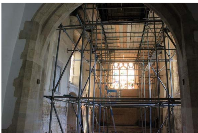
K Chancel interior scaffolded for ceiling lining and wall plaster repair. L Thomas Fisher’s sketch c1810 showing original pitched medieval roof line against the tower; its flatter pre-1866 successor is invisible below the level of the parapets.
