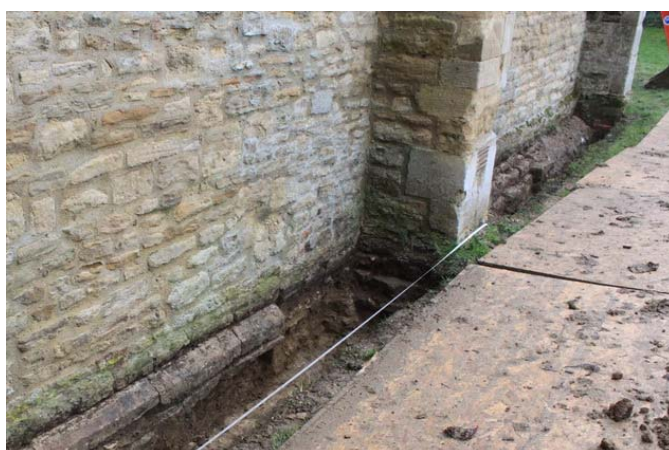
South side of chancel showing (left - C ) different stonework coursing on the doubled length to the right of the buttress, and (right - D ) in the drainage trenches the chamfered offset at a lower level on the original shorter chancel to left of the buttress.
