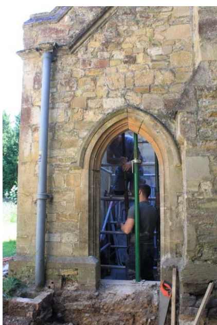
Vestry door enlargement: E before
