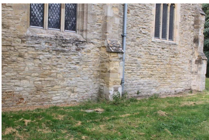
South side of chancel showing (left - C ) different stonework coursing on the doubled length to the right of the buttress, and (right - D ) in the drainage trenches the chamfered offset at a lower level on the original shorter chancel to left of the buttress.
