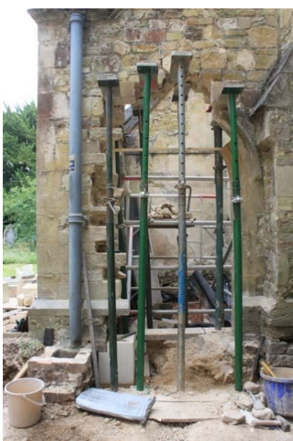
F propped during work
