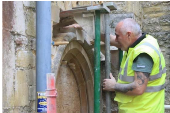
J easing the new keystone into position
