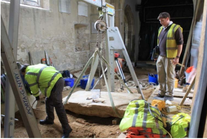
F Resettling a large ledger for reburial under the new floor
