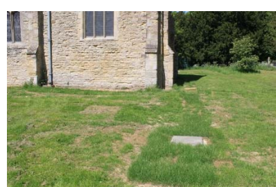
B Drainage north of chancel: footings exposed in trench; gravel-filled trench; drainage runs with soakaway in foreground; back-filled area.
