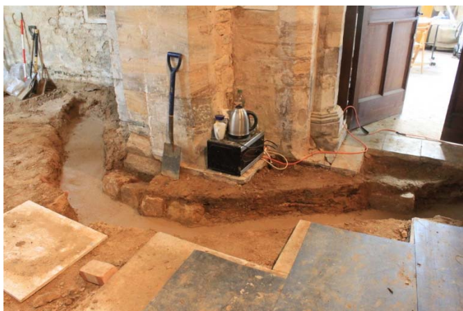
L Services channels running from the south transept (right) to the site of the future kitchenette (left)
