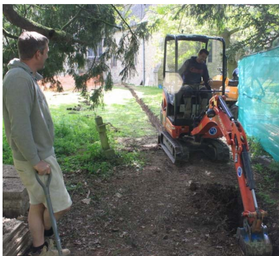
D Digging the modified shallow drainage to Coplowe Lane
