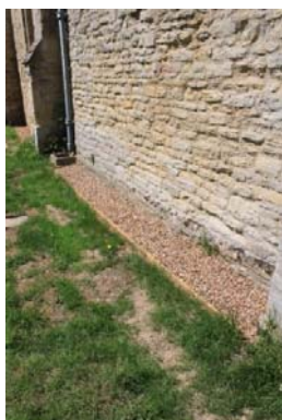
B Drainage north of chancel: footings exposed in trench; gravel-filled trench; drainage runs with soakaway in foreground; back-filled area.
