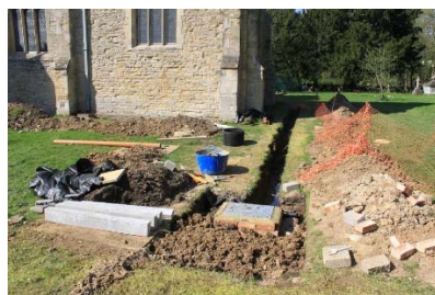
B Drainage north of chancel: footings exposed in trench; gravel-filled trench; drainage runs with soakaway in foreground; back-filled area.
