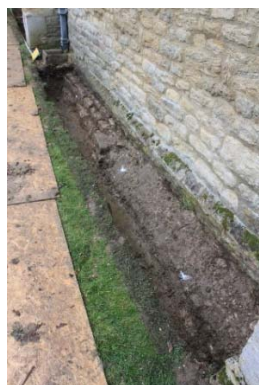
B Drainage north of chancel: footings exposed in trench; gravel-filled trench; drainage runs with soakaway in foreground; back-filled area.
