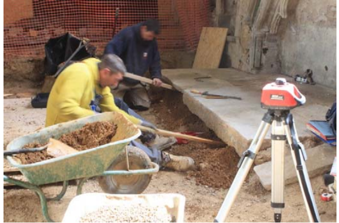
G Packing ground under ledgers retained for the new floor
