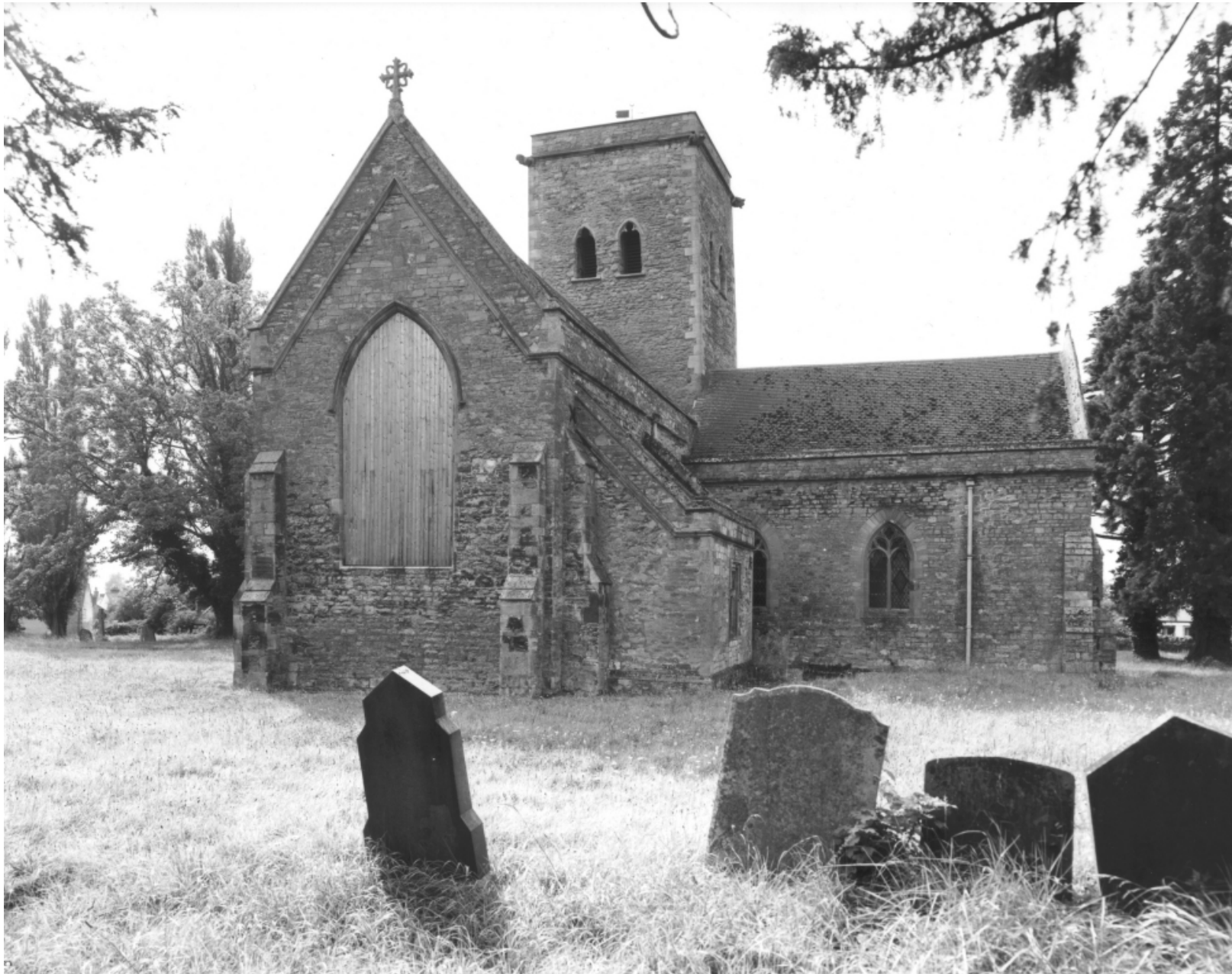
Chancel and North Transept, 1979.
