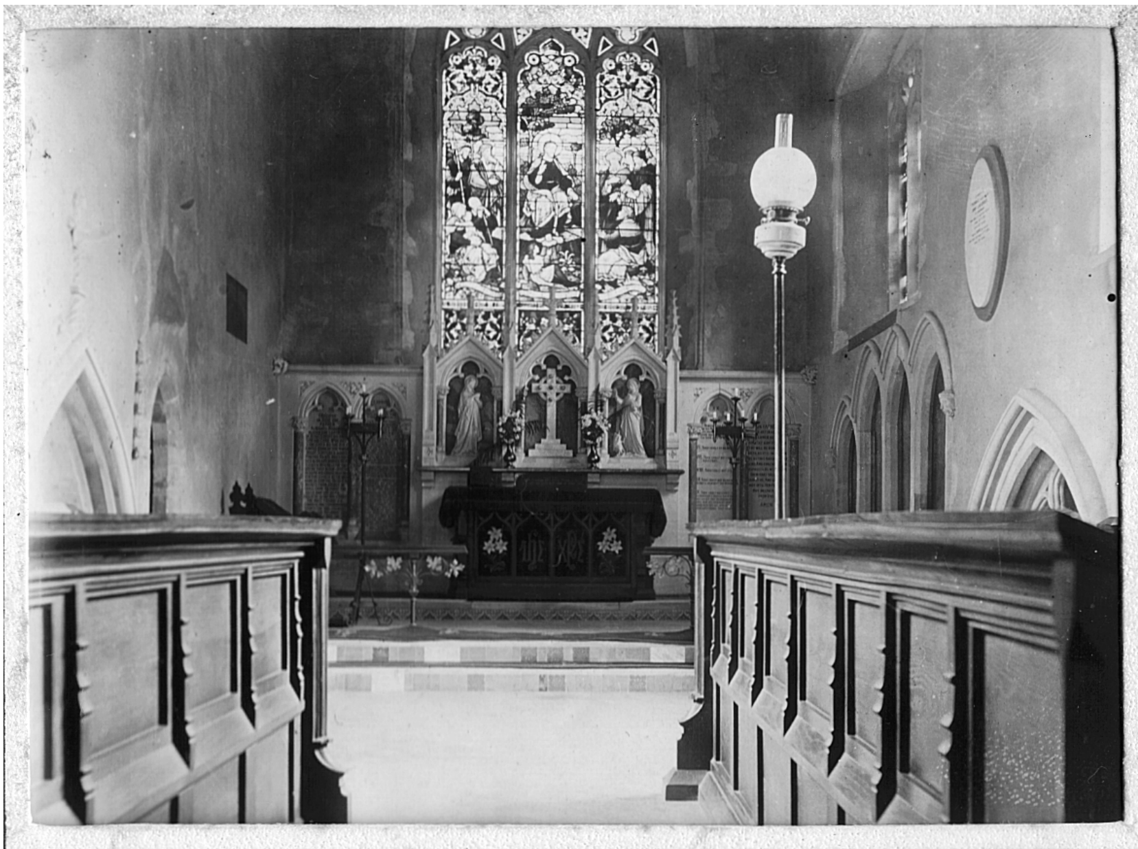
Chancel facing east c1907
