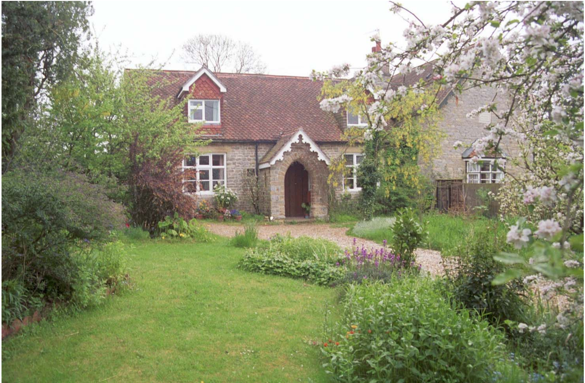
Old School & School House, Bletsoe 2000 EB233 ( David Baker )
