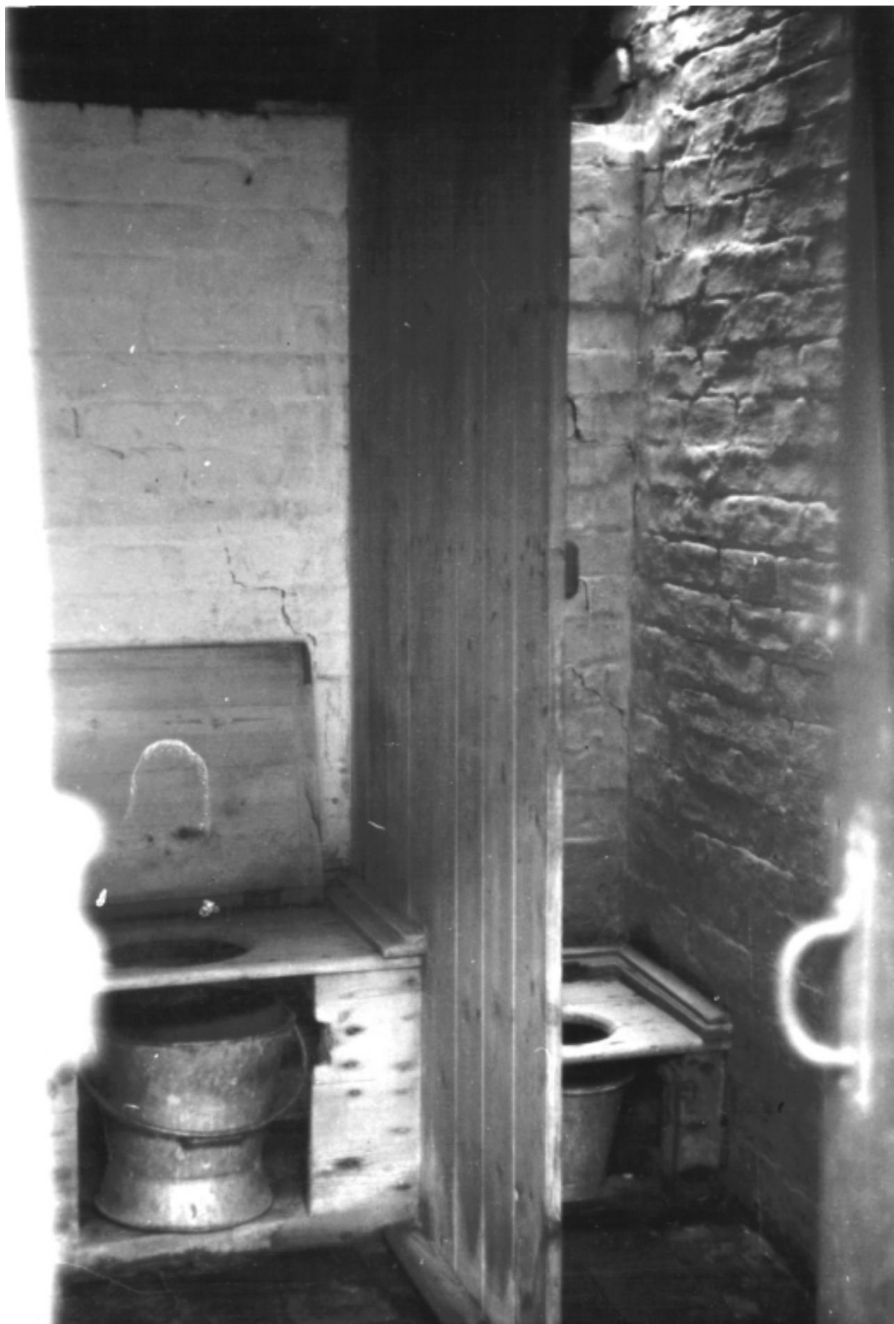
Sanitary arrangements at Bletsoe School, nd, possibly 1950s EB181 ( Bedfordshire Archives and Records Service Z55-1-21 )
